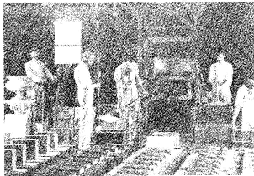
Illustration No. 83. Interior view of the Concrete Works (B-36) showing the manufacturing of the imitation "brownstones" used to face the first floor of the Founder's House. Photograph circa 1906.
